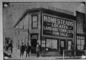
The old England block, one of the buildings to go up in smoke. At the time of the fire it was occupied by Clark's real estate agency, Mrs. Quantz' restaurant, and the government telephone office. At the right is Delong & May's general store, while to the left is shown the Great West hotel, which nearly was caught by the flames.
